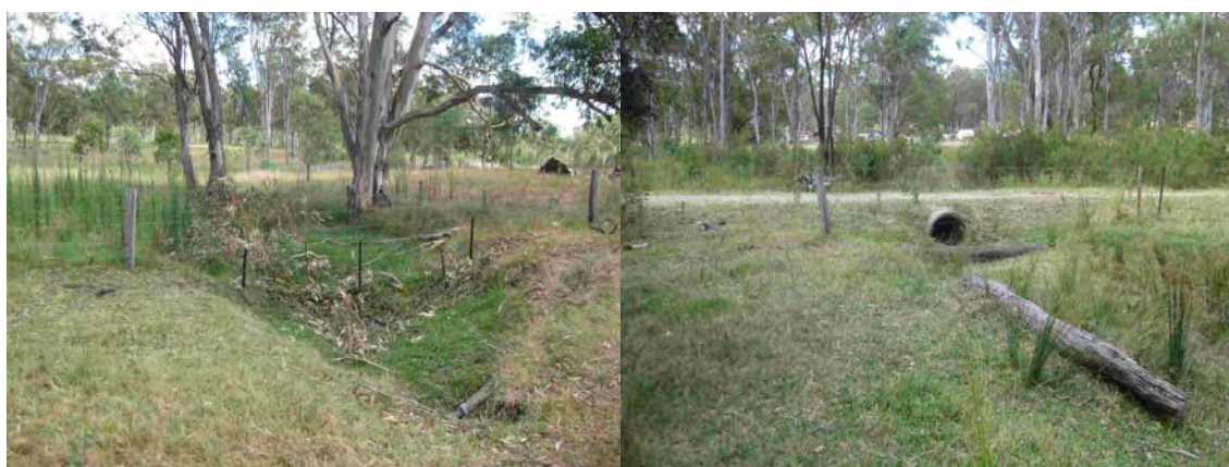
Photos 11 and 12 – Taken in the middle section of Tributary 2, near Basin 4. Photo 11 shows one of the many fence crossings. Fence crossings can capture debris which can cause localised scour of the channel. This is apparent in Photo 11 . Photo 12 shows one of the many culverted road crossings.
