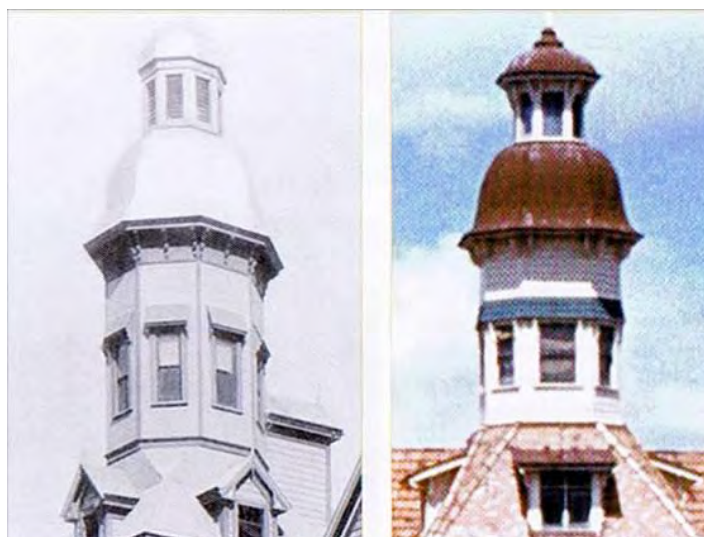
Figure 4.11 Original tower built 1903, rebuilt tower after the fire of 1919. Note the change in window form (Patrick 2003:25).
