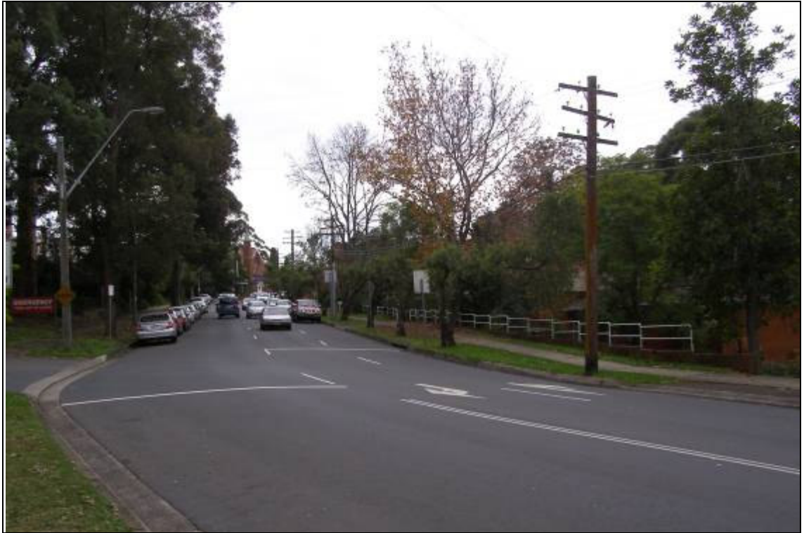
Photograph B.001 -- Above ground electrical cables in Fox Valley Road
