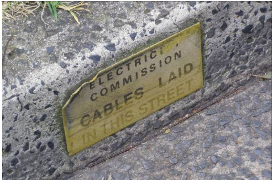
Photograph B.002 - Electrical cables in Fox Valley Road verge-
