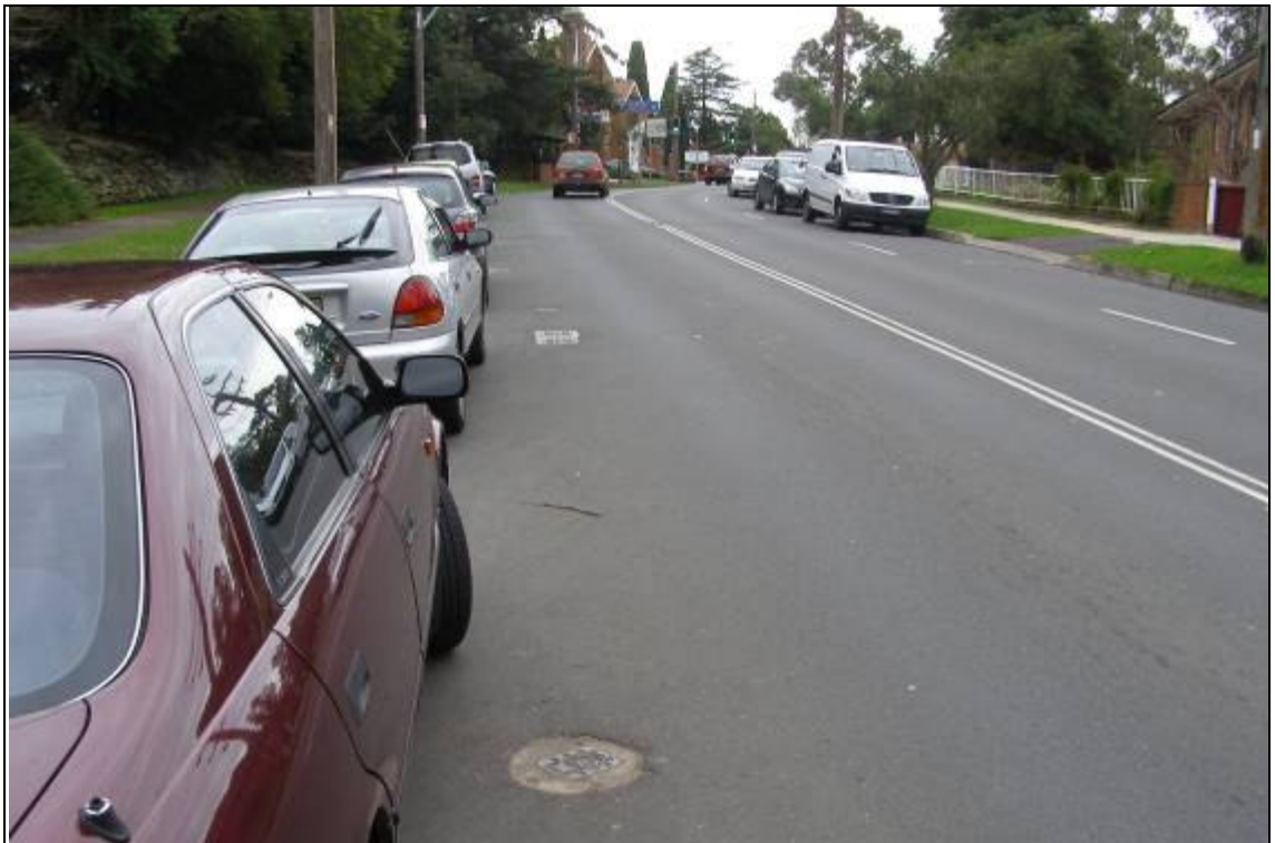
Photograph B.004 - Water main in Fox Valley Roadway-
