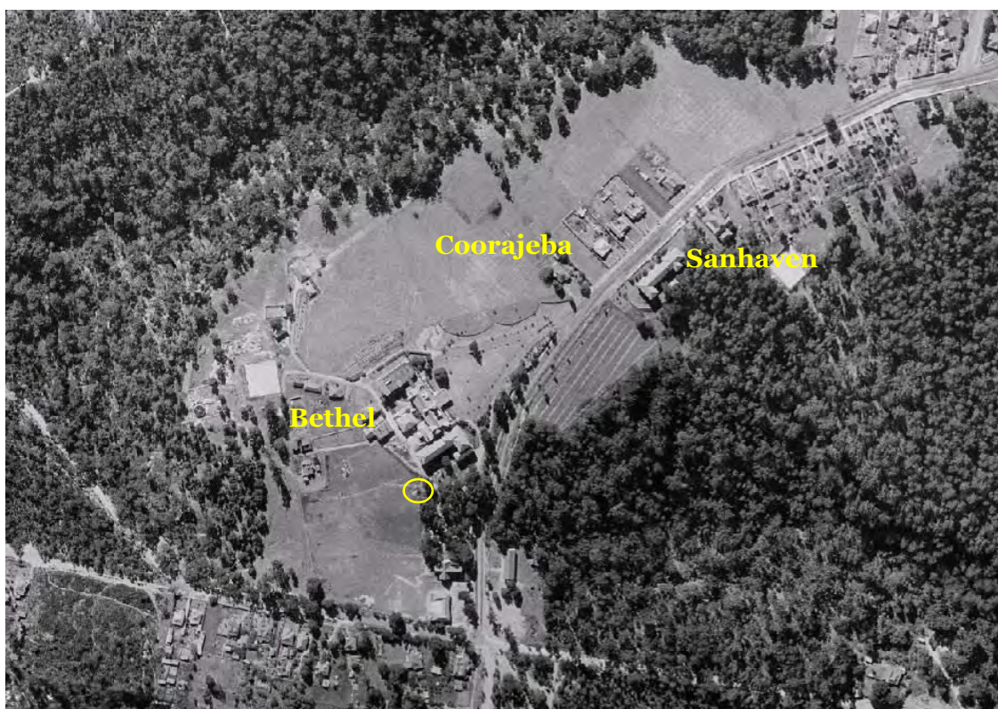
Figure 4.31 1943 aerial showing Bethel, Coorajeba, Sanhaven and a tentative location for the nightwatchman's shelter (circled)
