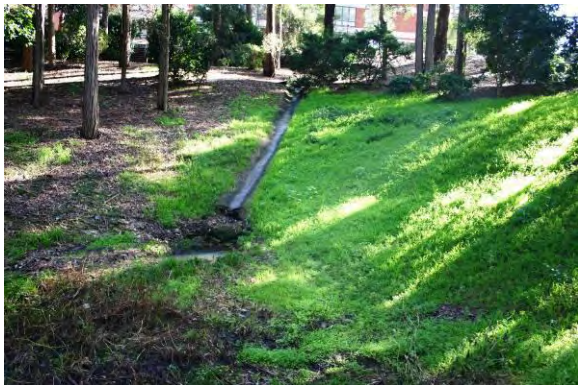
Concrete drain into depression behind Administrative Headquarters building
