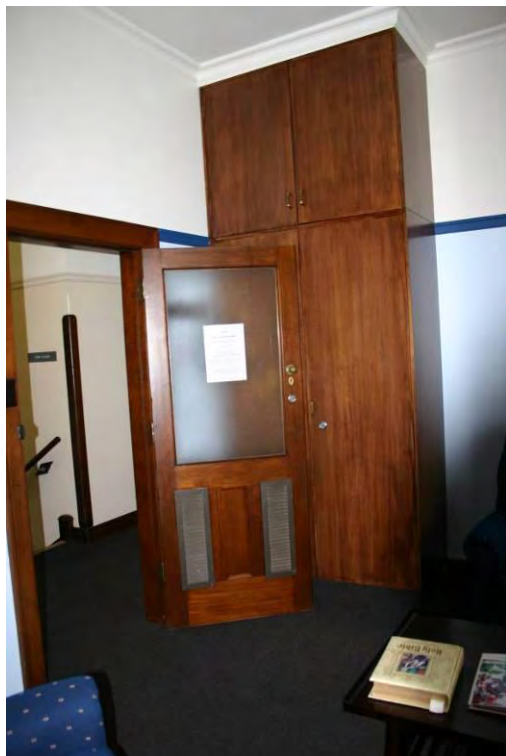
Original timber detailing of built-ins and fittings
