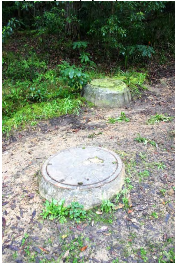
Service access hatches near creek
