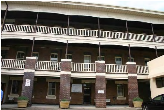
The west front elevation of the Shannon Wing. The removal of the balcony from the north elevation is demonstrated by the exposed balcony joists (arrowed right).
