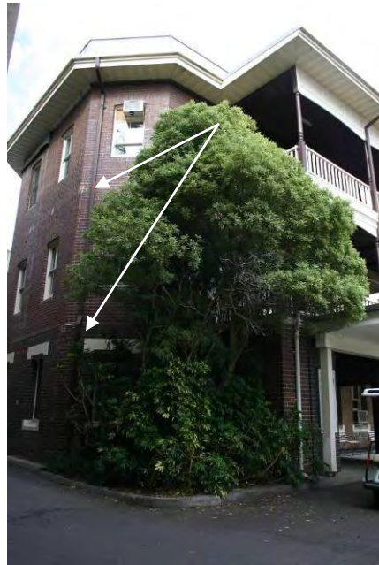
The west front elevation of the Shannon Wing. The removal of the balcony from the north elevation is demonstrated by the exposed balcony joists (arrowed right).
