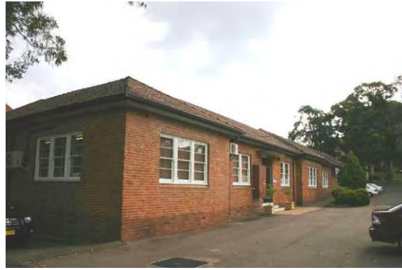
School building northeast corner
