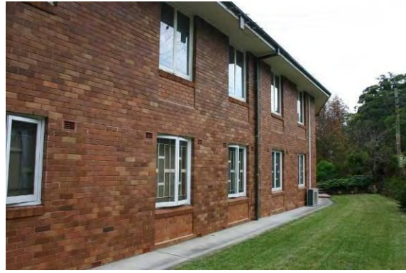
Ladies Hostel west elevation detail
