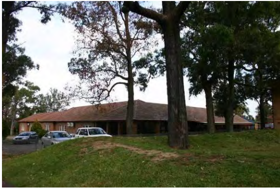
School building east elevation
