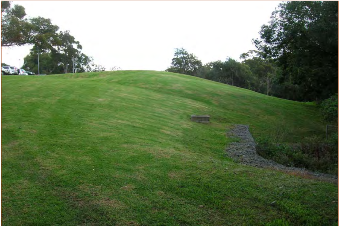
PHOTO 6: Filling at edge of carpark
