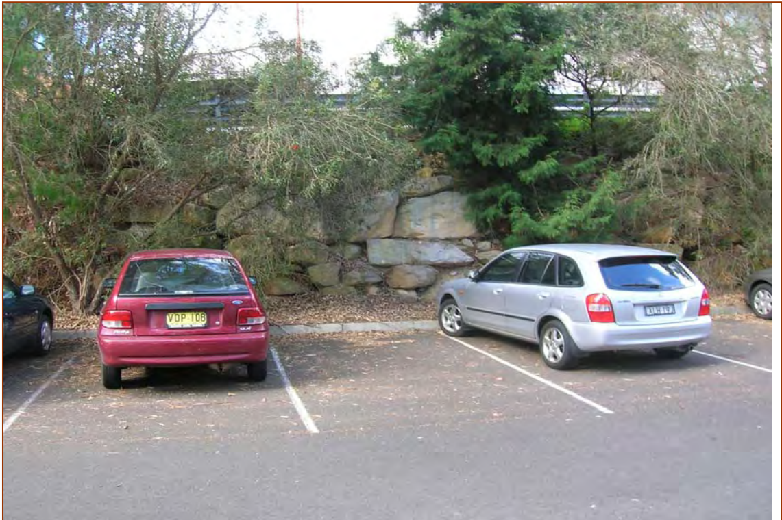
PHOTO 10: Sandstone Block Retaining Wall
