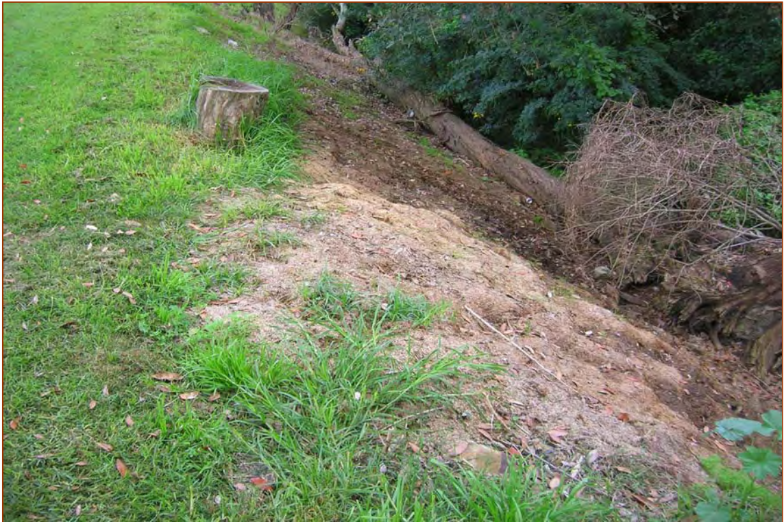
PHOTO 8: Filling near edge of carpark
