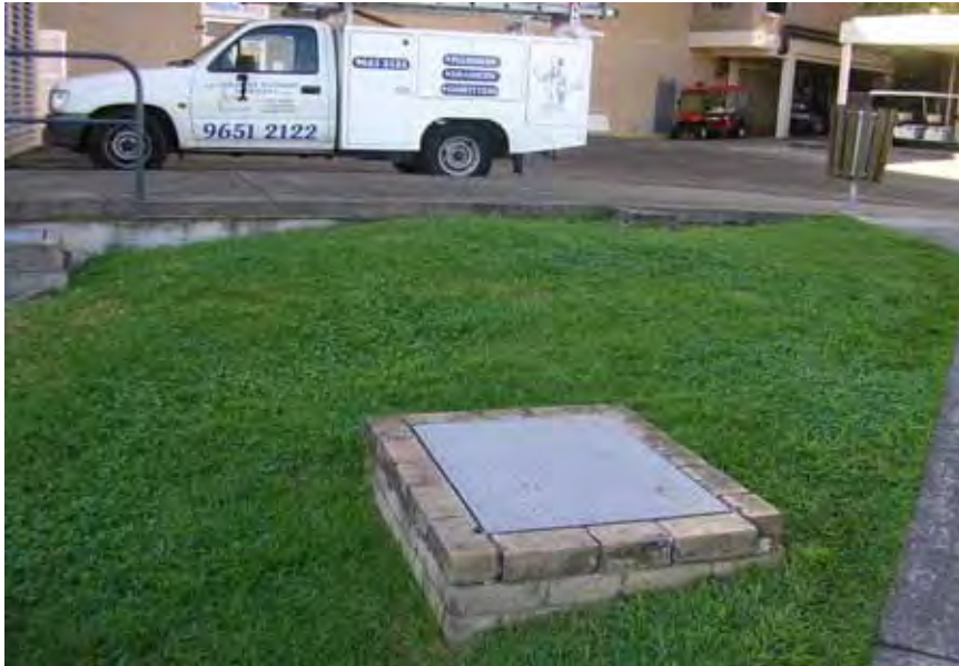
Photo 11: Underground fuel storage tank (UST) DG 15
