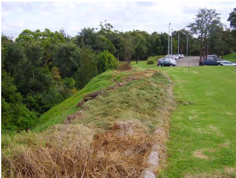
Photo 2: Looking west along the fill batter slope located immediately south of the proposed Building 3 southern boundary. The slope was covered with grass cuttings and overgrown vegetation with fragments of brick and concrete also noted
