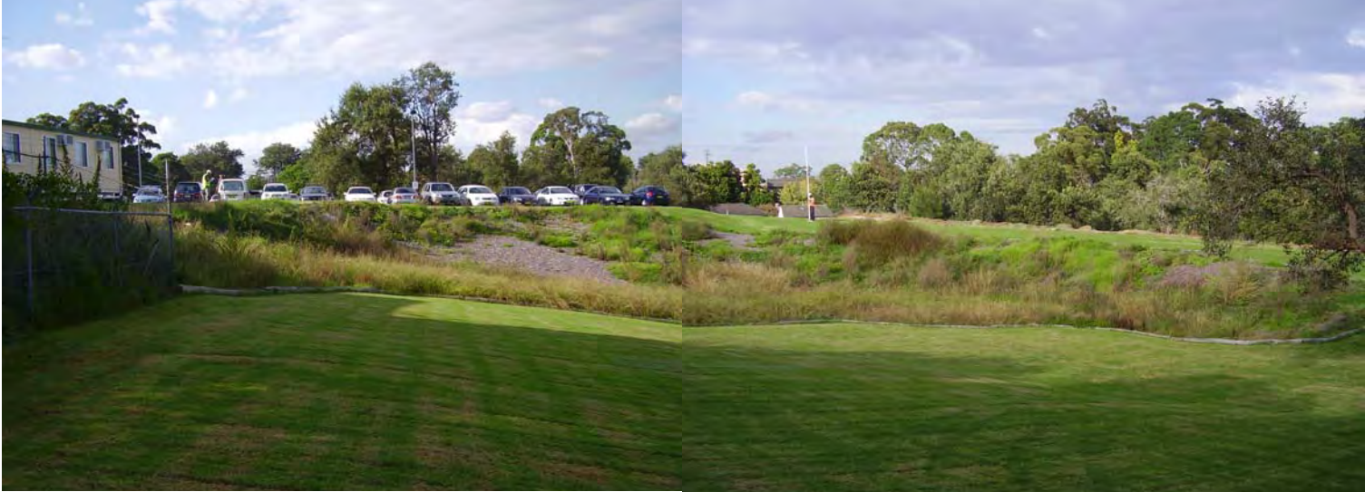
Photo1: Looking east from the north western corner of the proposed Building 3 towards the retention basin centrally located within the study area
