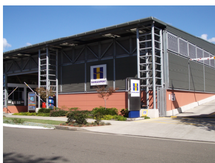
Figure 29: Overhanging eaves, louvres & distinctively detailed structural elements
