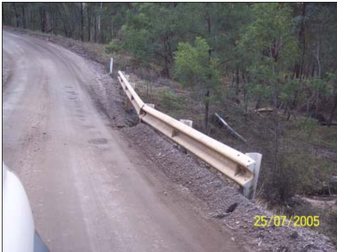
VIEW OF BOX CULVERT HAZARD AT CH 10.22 FROM RESORT WITH INADEQUATE GUARD RAIL PROTECTION
