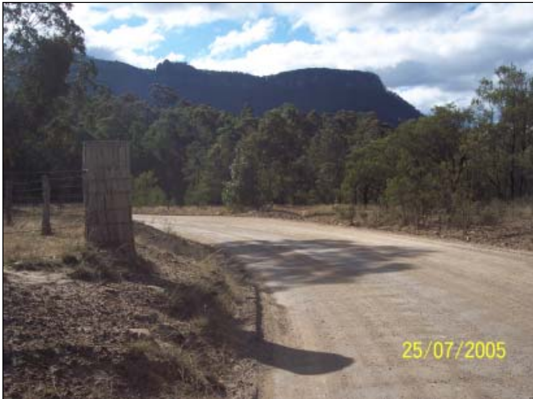
VIEW OF ISOLATED SPOT HAZARDS WITHIN THE CLEAR ZONE (TREE STUMP)
