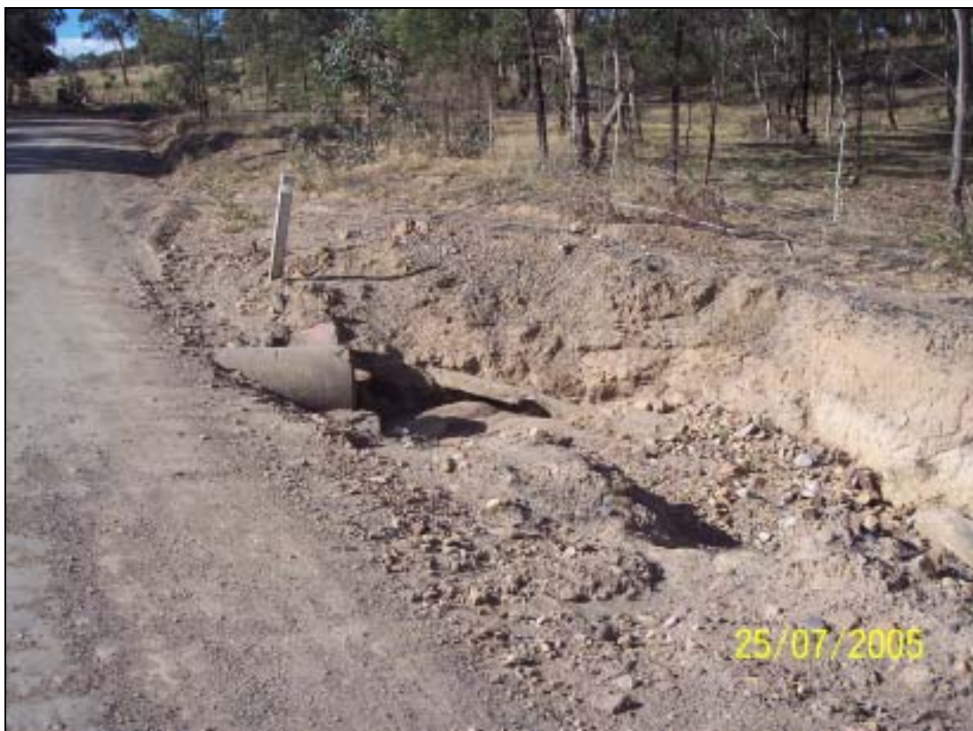
VIEW OF LOCALISED EROSION ALONG ROAD SHOULDER
