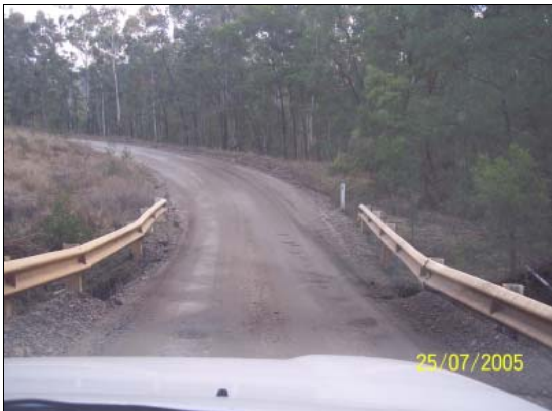
VIEW OF BOX CULVERT HAZARD AT CH 10.22 FROM RESORT WITH INADEQUATE GUARD RAIL PROTECTION
