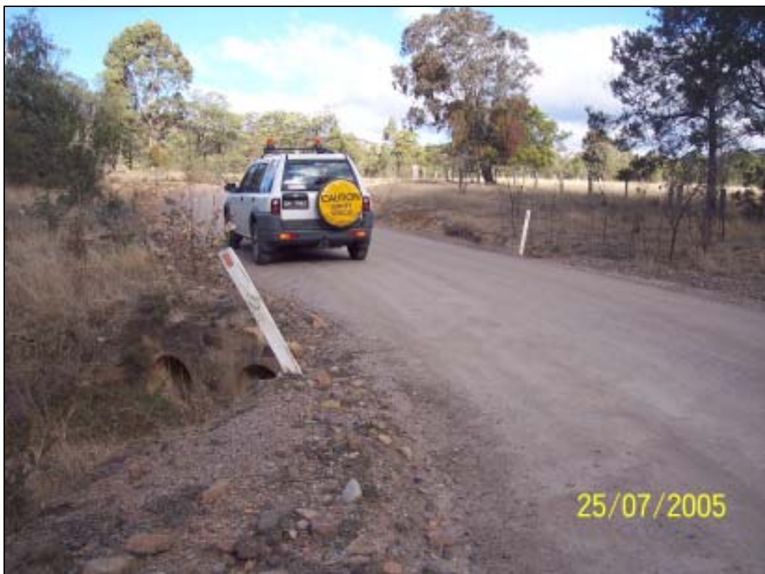
VIEW ISOLATED SPOT HAZARDS WITHIN THE CLEAR ZONE (EXPOSED CULVERT)
