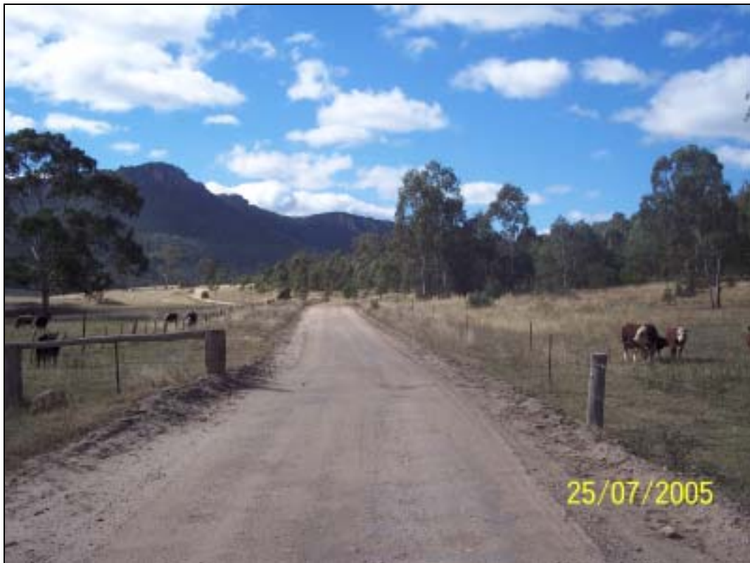
VIEW OF ISOLATED SPOT HAZARDS WITHIN THE CLEAR ZONE (FENCE POST)
