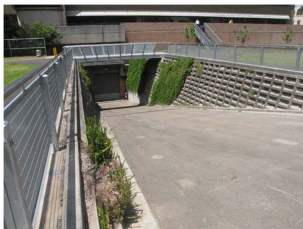
Figure 5.6 Looking south down the basement access road, demonstrating the extent of cutting into soil deposits. (Source: GML)
