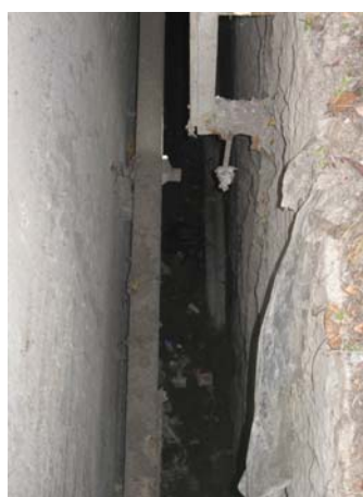
Figure 5.8 Looking into the cavity between the edge of the UTS tower (on the left) and the cutting in the surrounding bedrock (on the right). (Source: GML)
