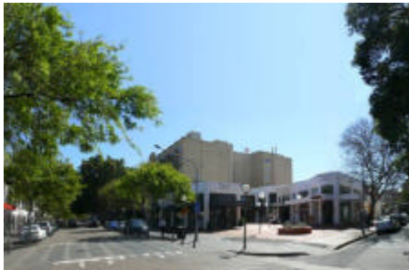
Figure 28 View 12 – Corner of Cross Street and Transvaal Avenue The existing building presents a blank, poorly articulated wall to the corner of Cross Street and Transvaal Avenue.
