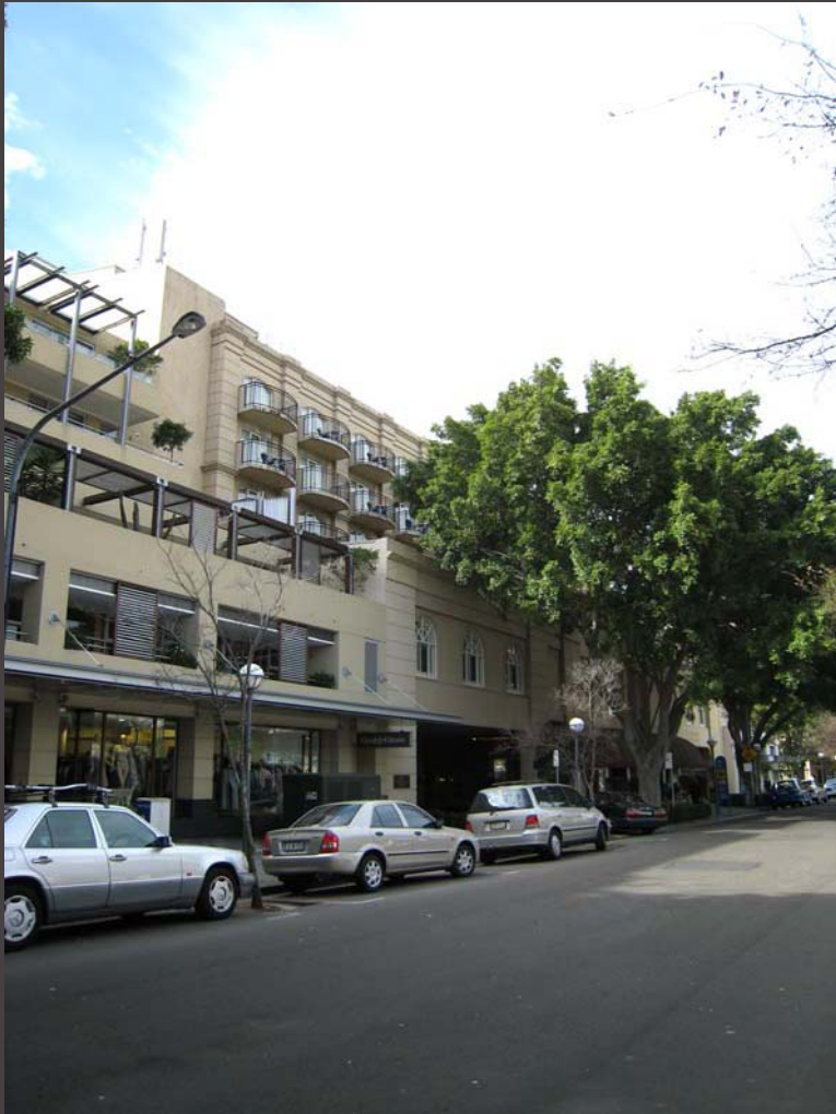
View from Cross St looking East - Existing trees largely screen building bulk
