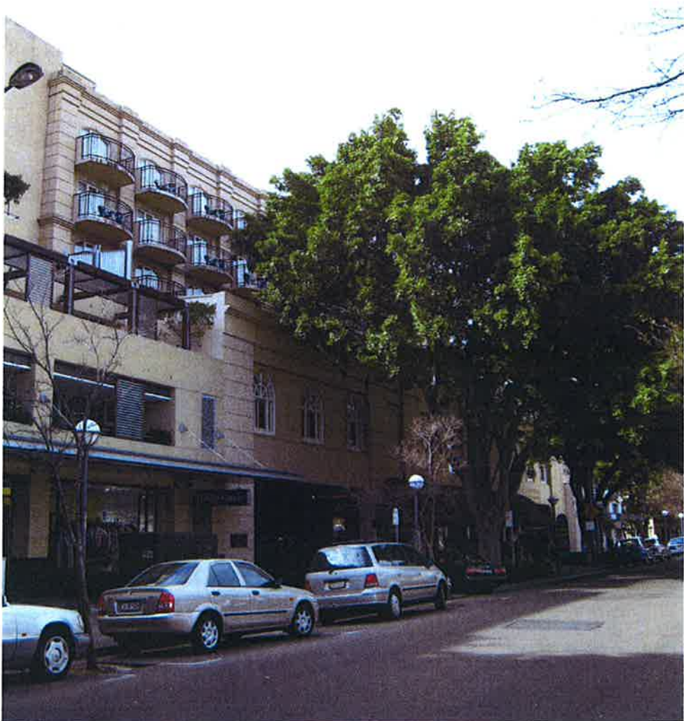
FIGURE 1.2 - The Stamford Plaza Hotel, 33 Cross Street, Double Bay
