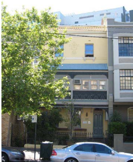
The front elevation of 372 Victoria Street.
