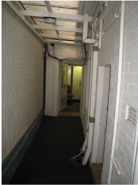
Corridor linking the front and rear buildings.
