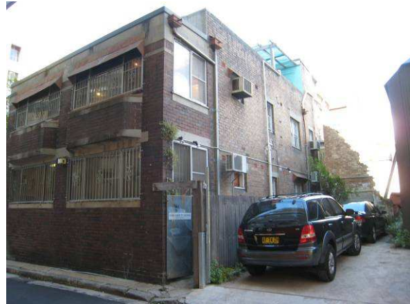
The c1931 addition to the rear of the site.
