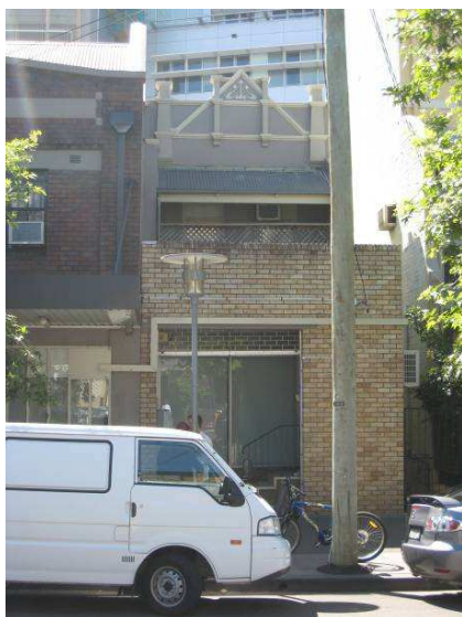
Figure 15 – Photograph of 370 Victoria Street
