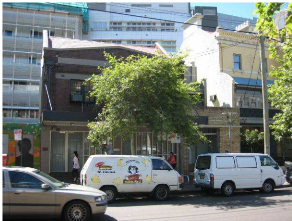
Figure 14 – Photographs of 366-368 Victoria Street
