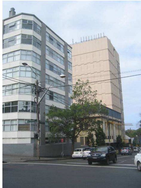
The Telstra Exchange Building (right) – Liverpool Street.
