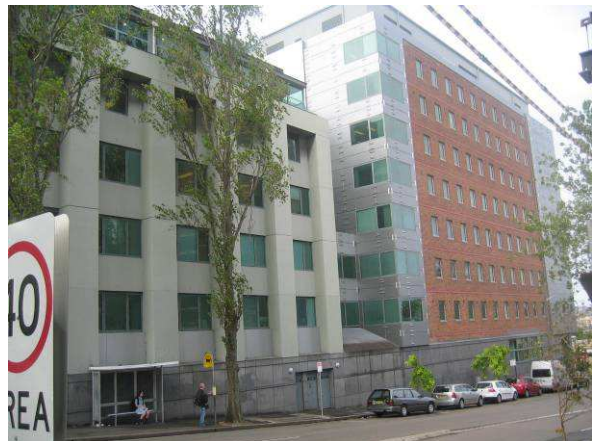
Garvan building in Burton Street.
