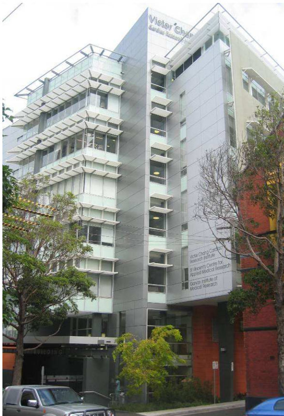
Victor Chang building, 405 Liverpool Street (corner of Chaplin Street)
