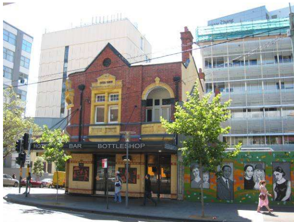
Green Park Hotel, 360 Victoria Street (not part of the site) with Victor Chang building (405 Liverpool Street) in the background (right).
