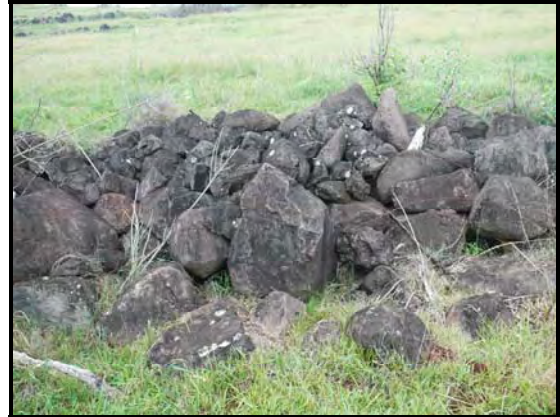
Figure 22 – Example of a substantial boulder retaining wall
