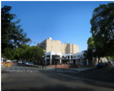
Figure 35 View 13 – Corner of Cross Street and Transvaal Avenue
