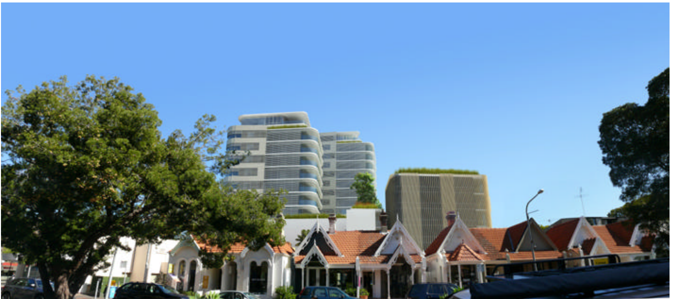
Figure 73 Proposed view from Transvaal Avenue, Double Bay (looking directly at site)
