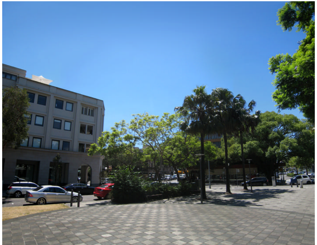
Figure 78 Existing view from Guilfoyle Park
