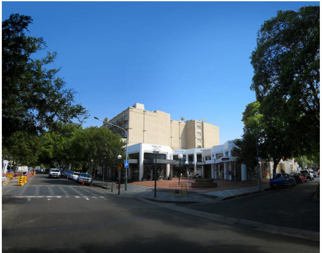
Figure 68 Existing view from the corner of Cross Street and Transvaal Avenue
