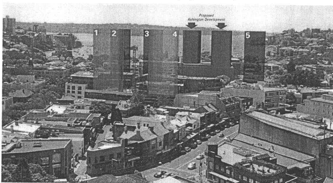
Fig 1: Potential development scenario if 15 storey development precedent is set by Ashington proposal
