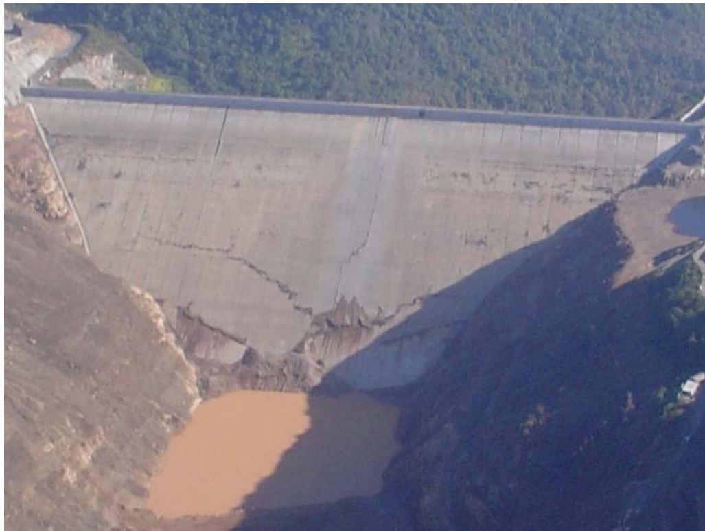
Figure 7-2 - Compression Failure in Face Slab at Campos Novos Dam
