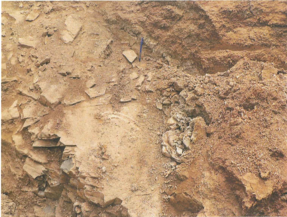
Plate TF7. Chn.19.5m. Fault plane dipping downstream.
