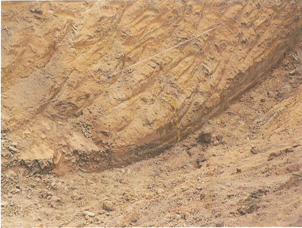
Plate TF3. Chn.17m to 22m. General view of the fault plane dipping downstream (to the right of the photograph).
