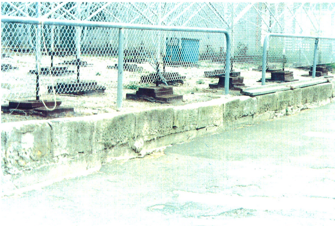
Figure 3.1d Visual Inspection: Retaining wall of re-used sandstone at base of Giant Slide - site of Busby's Bore located in 1974 (outside re- development area).
