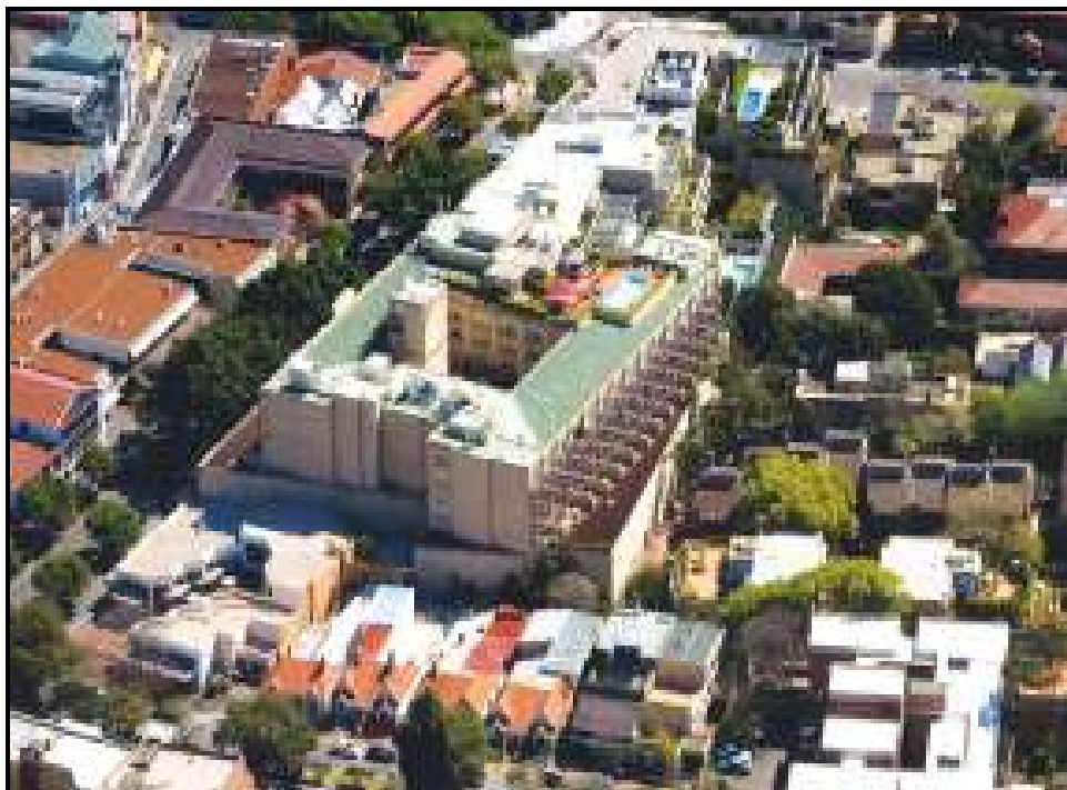
Photograph 1 - Aerial view of the existing Stamford Plaza Hotel building
