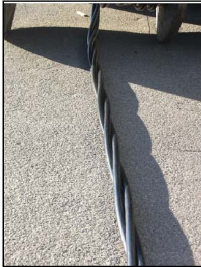
Fig. 17a 11kV XLPE insulated cable in Triplex arrangement
