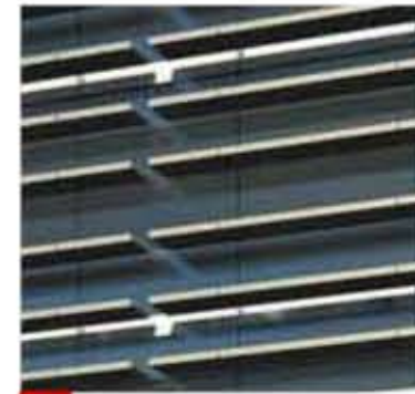
FLOOR TO FLOOR GLAZING BEHIND SUNSCREEN
