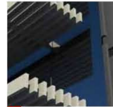
ANODIZED ALUMINIUM HORIZONTAL SUNSCREEN
