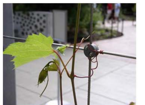
Detail of stainless steel climbing frame
