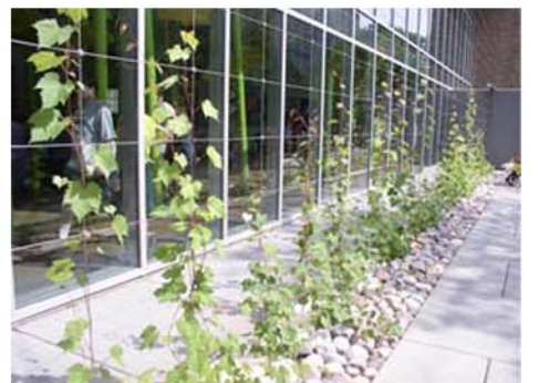
Climber on stainless steel rod frame
