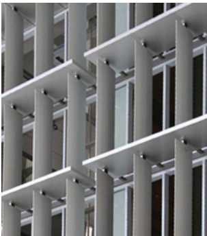
ES2 - EXAMPLE OF EXTERNAL SUNSHADE - FIXED ALUMINIUM BLADES/FRAME
