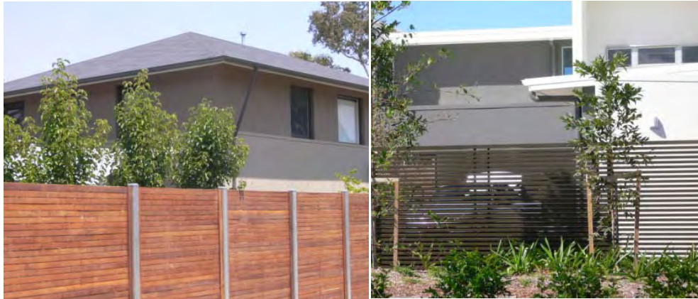
Figure 3.1.9.4: Examples of translucent fencing on a secondary boundary of a corner site
