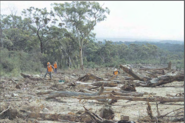
Photograph 3 Re-spreading of vegetation over easement through Moreton National Park, NSW.
