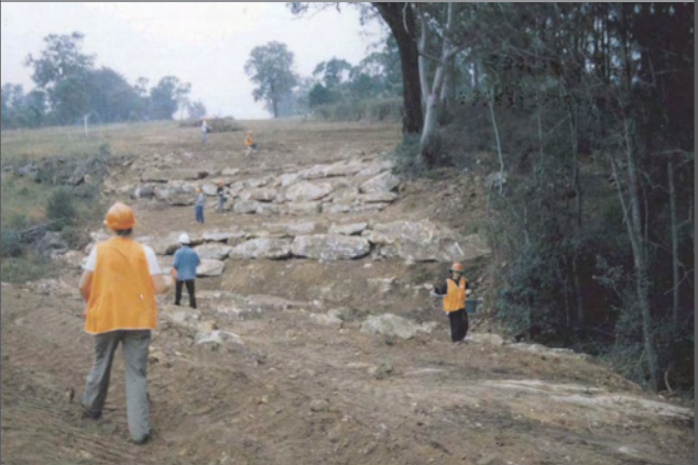
Photograph 6 Hand-broadcasting of seed along drainage line. Rock walls placed to assist with bank stability.
