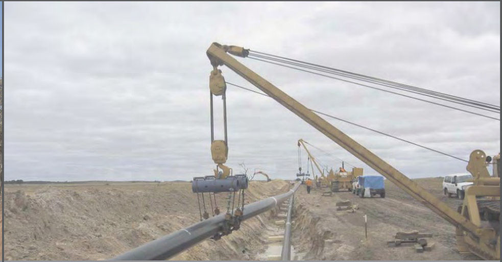
Photograph 6 Lowering in of pipe
