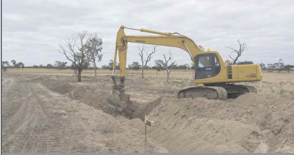
Photograph 7 Backfilling of trench following lowering of pipeline
