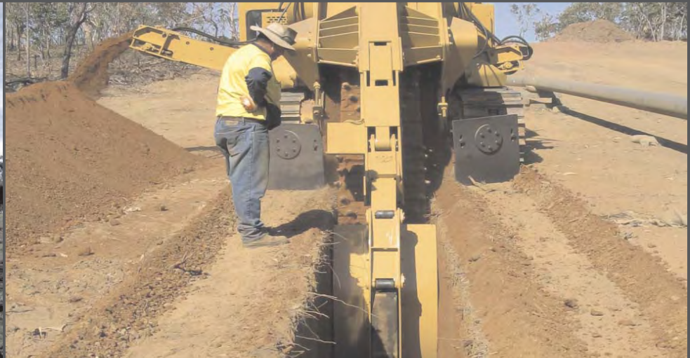
Photograph 4 Trenching using trenching machinery
