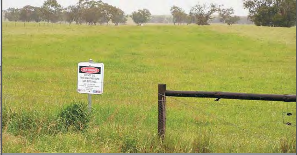
Photograph 8 Reinstatement of ROW including pipeline marker
