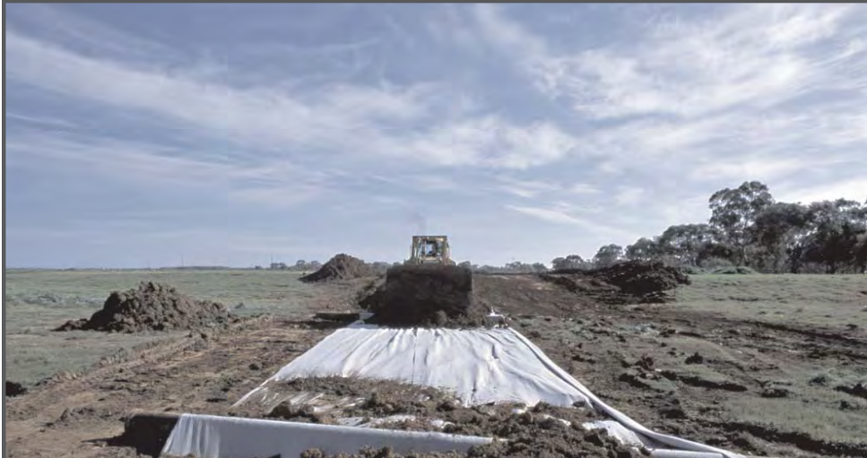
Photograph 3 Grading and stockpile preparation including placement of drainage pipe to allow runoff to drain through stockpile
