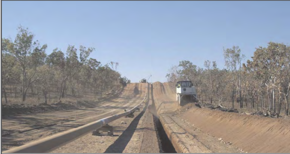
Photograph 5 Padding of pipe trench prior to lowering of pipe
