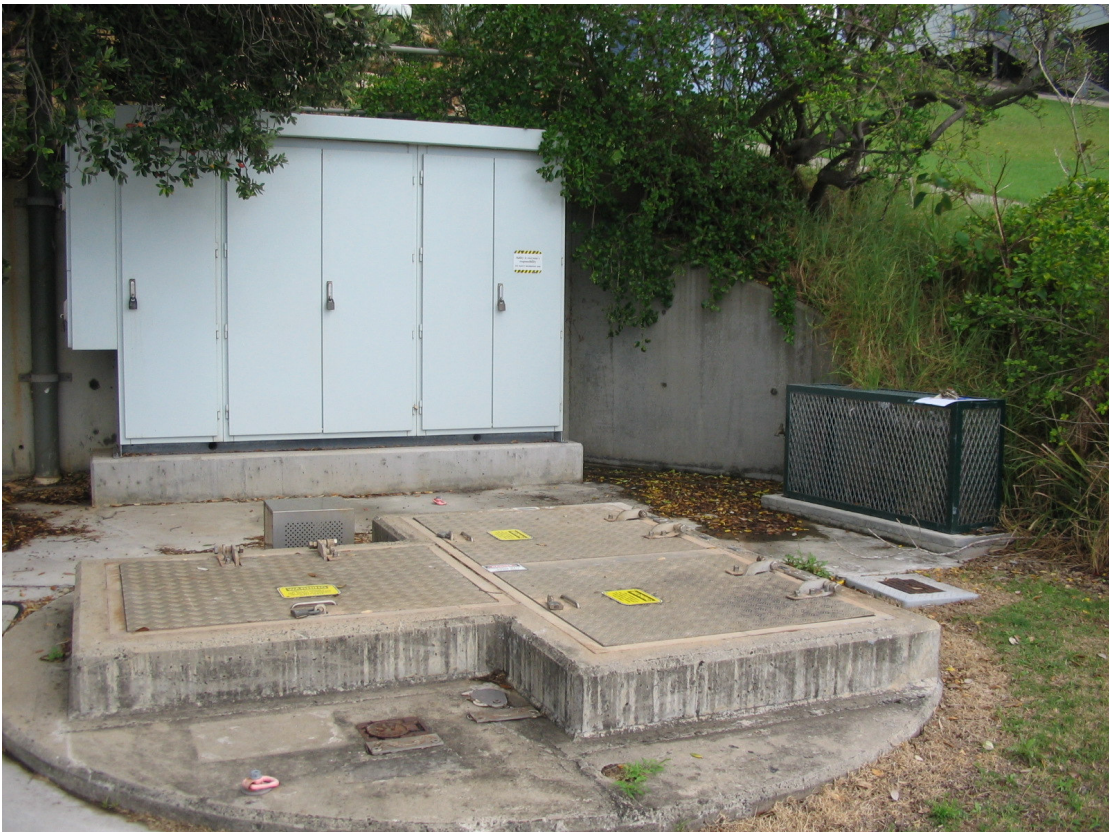
Figure 6 Typical small wastewater pumping station
