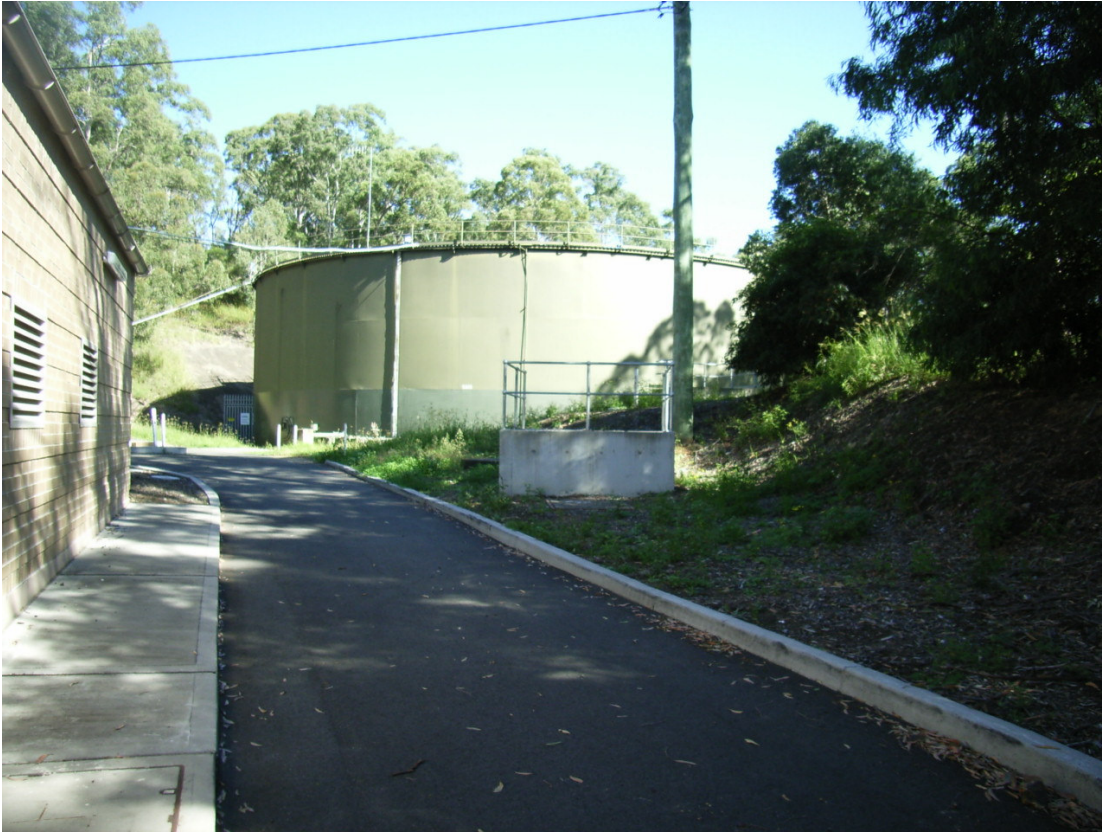
Figure 4 Typical surface reservoir
