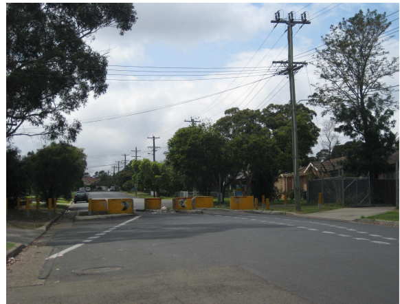
Picture 8 – Traffic management works to prevent heavy vehicle movements to east along Pavesi Street
