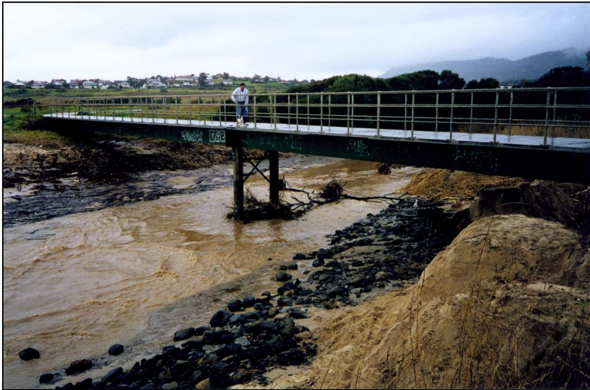
Figure 5 Photograph of Scour in Hewitts Creek Just After August 1998 Flood
