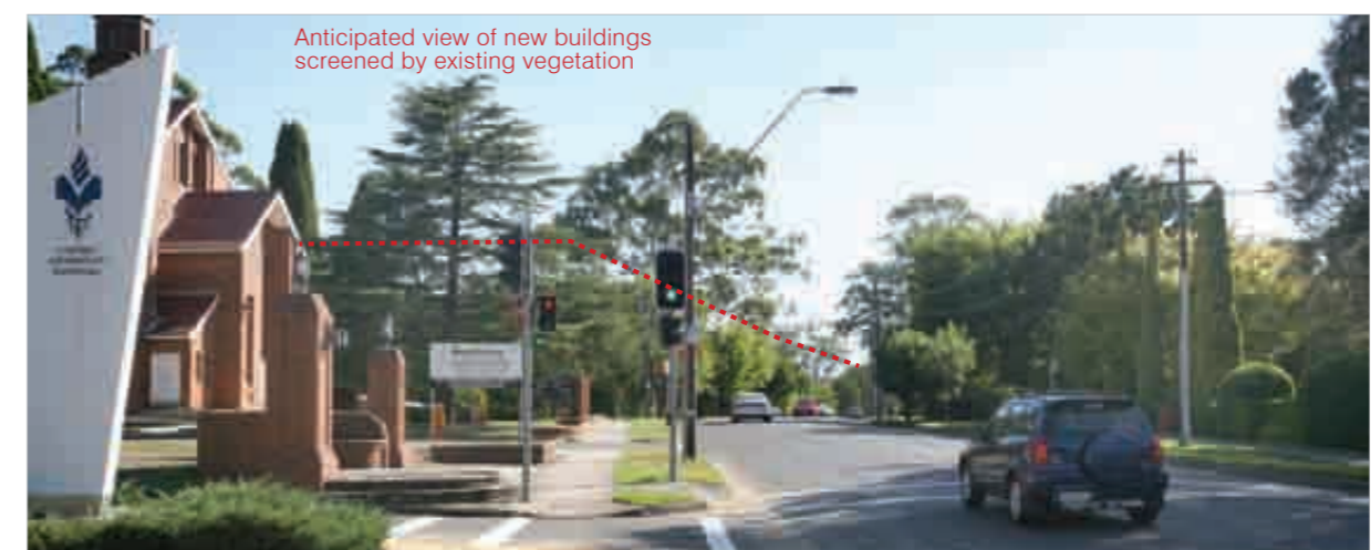
Figure 92 – View 1: Looking north along Fox Valley Road from main entrance to hospital
