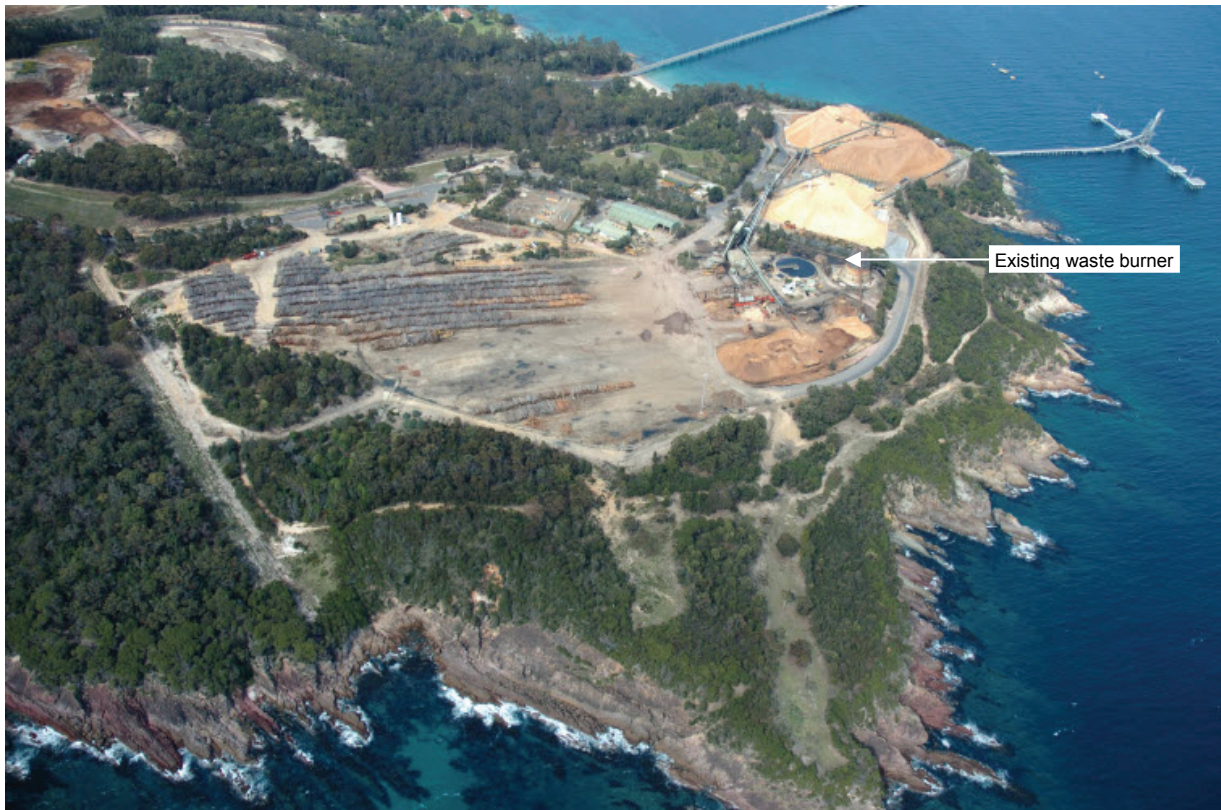
Figure 2-1 SEFE Munganno Point Mill Site
