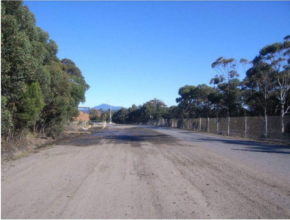
Plate 4. Route of proposed water transfer system from power plant to wharf. Photo taken adjacent to waste burner (to NNW) looking 240°. The two water pipelines will be installed on concrete blocks adjacent to the security fence.
