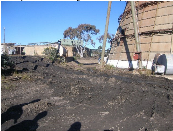
Plate 9. The area in which the mill waste burner is situated; note excavation.
