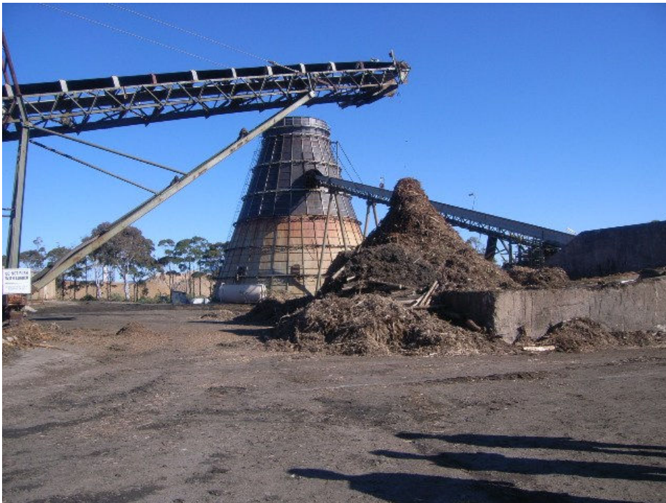
Plate 3. Looking from the storage area towards the waste burner site.
