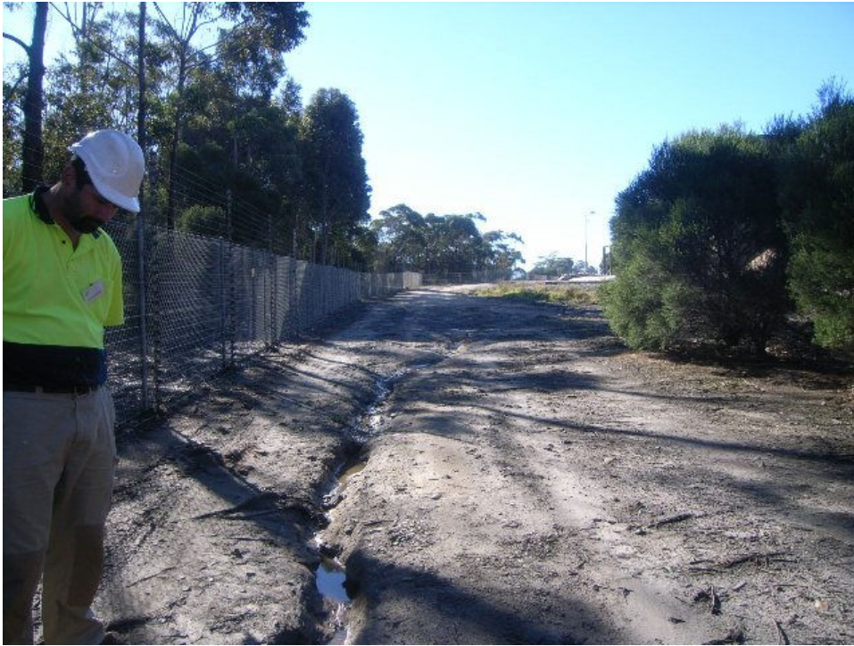
Plate 8. Route of proposed water transfer system from power plant to chip wharf. Photo taken at south end of a minor track looking northeast; note high erosion to clay.
