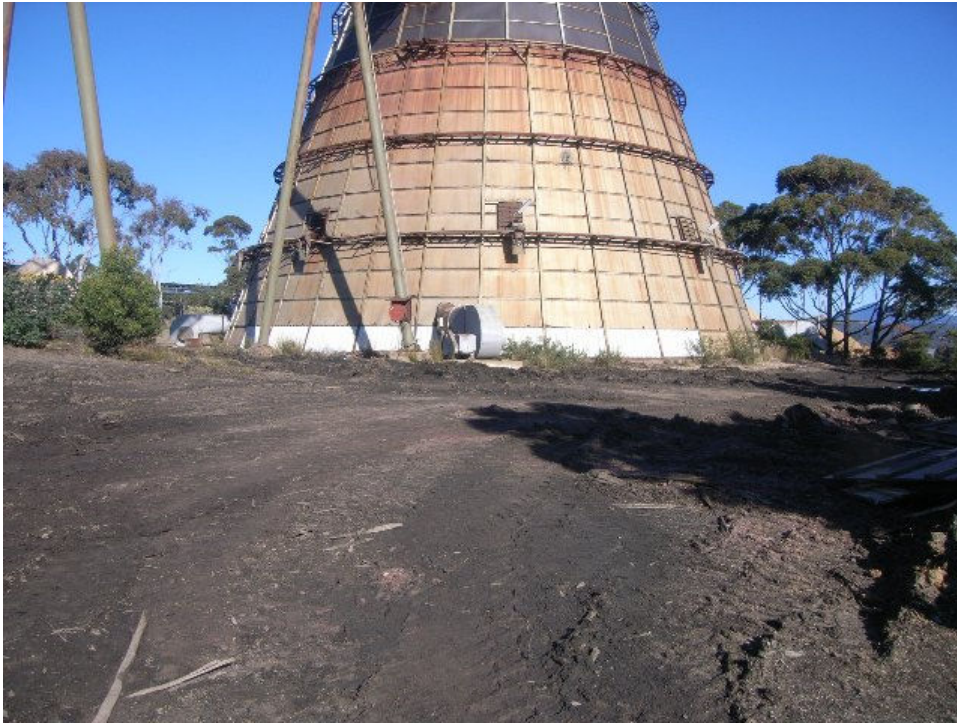
Plate 1. The mill waste burner site in which the proposed power plant will be situated.
