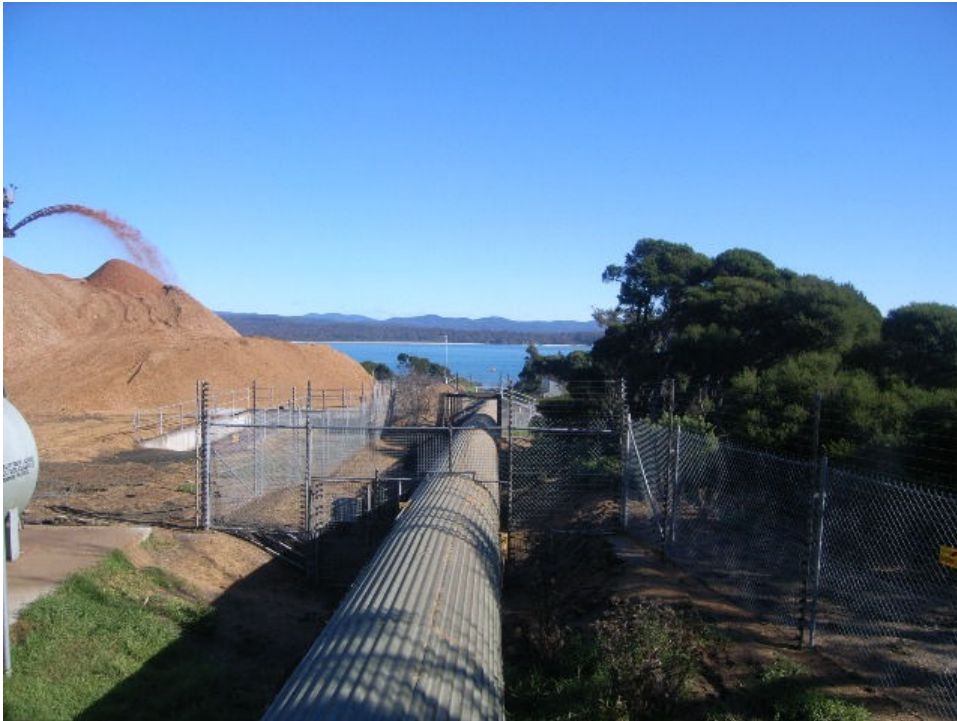
Plate 7. Route of proposed water transfer system from power plant to chip wharf. In this area the pipework will be attached to the existing conveyor which extends to the wharf. Photo taken at point where pipework will be attached to conveyor; looking northwest.
