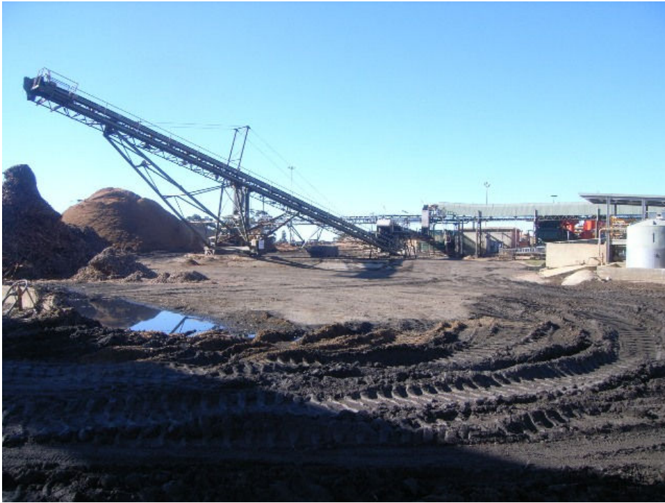
Plate 2. Existing storage area located adjacent and to the northeast of the waste burner.
