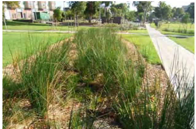
Bio stormwater bio swale
