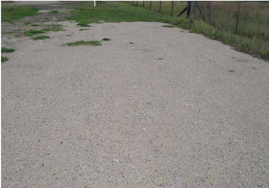
Photo 5: Recycled concrete backfill in former UST pit
