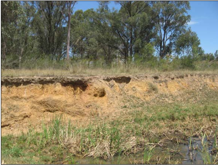
Figure 16. Indicative section of the excavated creek diversion channel in the vicinity of Site #45-5-0786 showing the lack of original topsoil and highly eroded nature of the channel.
