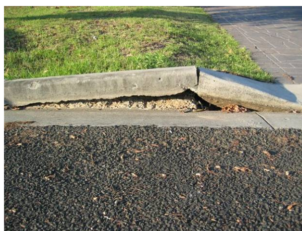
Fig. 5.3 Cracking and Buckling of Kerb at Tahmoor
