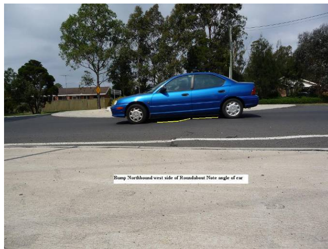
Fig. 5.2 Cracking and Bump at Roundabout at Tahmoor
