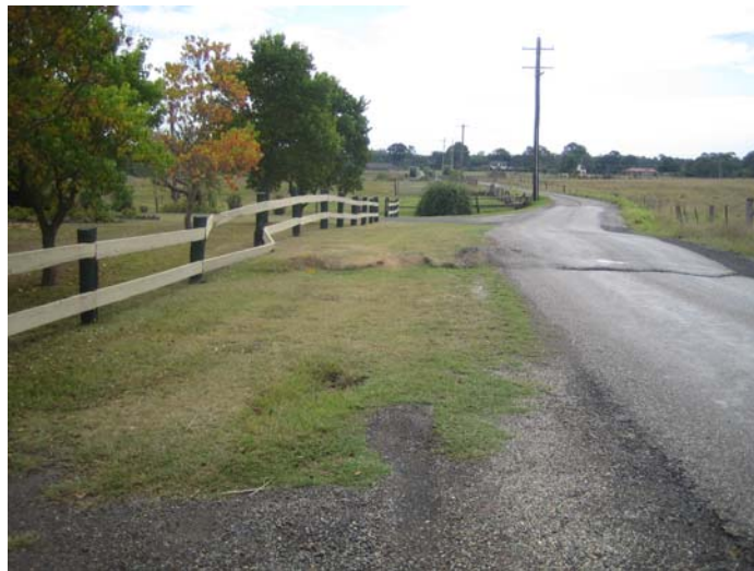
Fig. 4.10 Example of Surface Compression Humping along Outcropping of a Low Angle Thrust Fault
