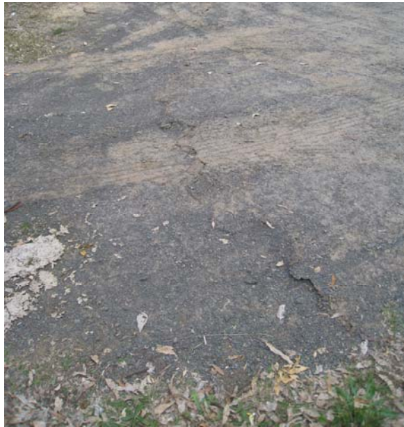
Fig. 4.11 Example of Surface Compression Buckling Observed in a Pavement
