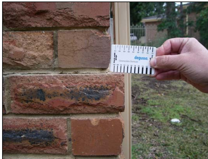
Fig. C.1 Example of slippage on damp proof course
