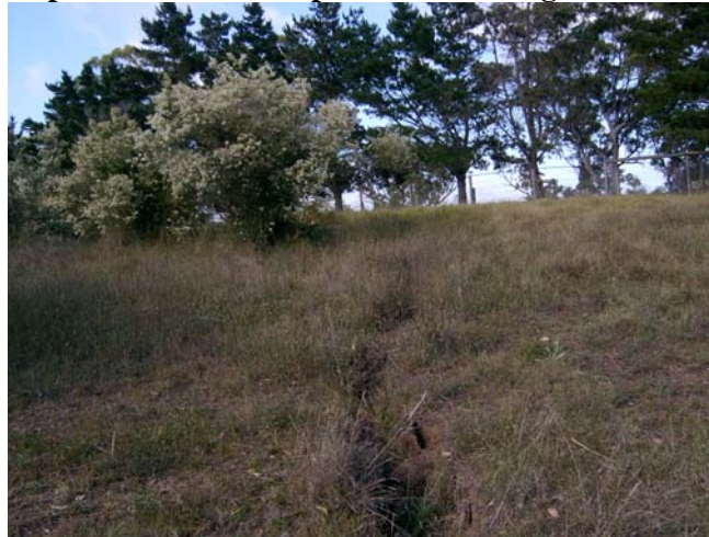
Fig. 4.12 Example of Surface Tension Cracking along the Top of a Steep Slope
