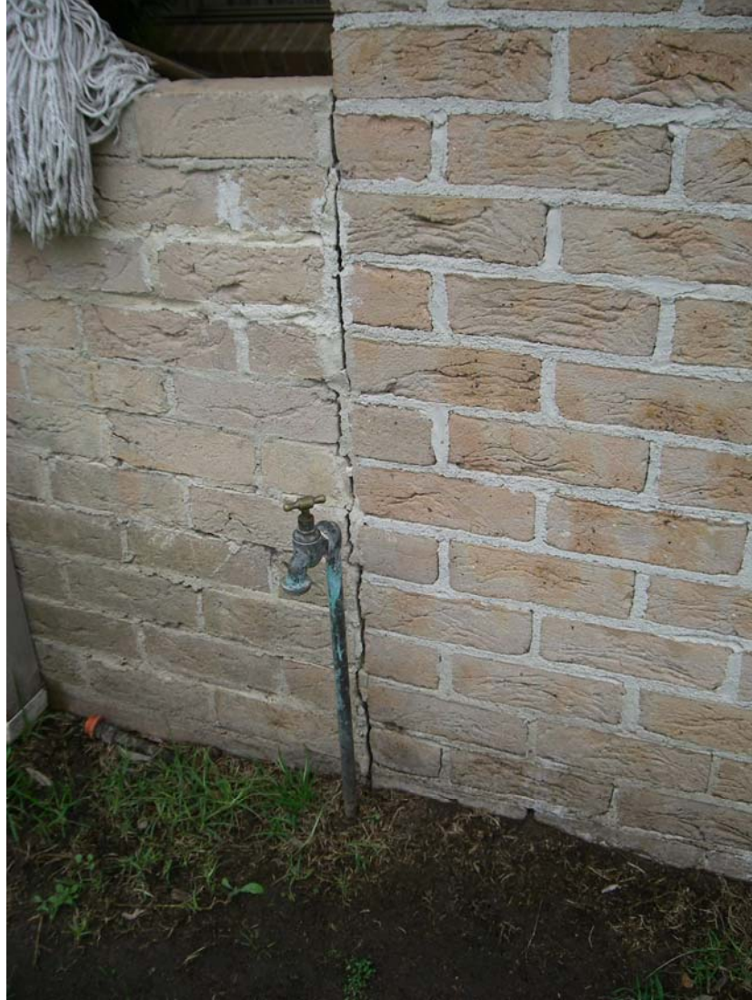
Fig. C.2 Example of crack in mortar only
