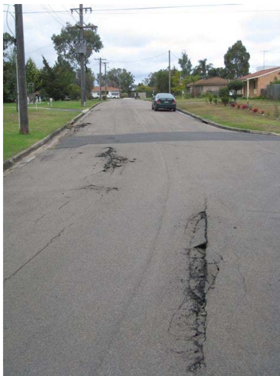
Fig. 5.2 Cracking and Bump at Roundabout at Tahmoor
