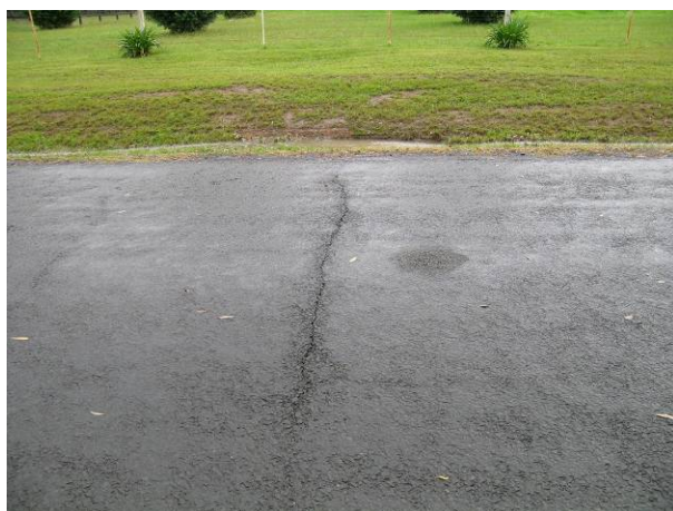
Fig. 5.3 Cracking and Buckling of Kerb at Tahmoor
