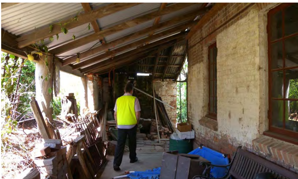
Figure 28 The skillion roofed annex to the barn showing the bush pole posts and the more recent sawn timber roof structure. Source: Paul Davies Pty Ltd November 2009.
