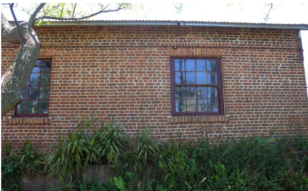
Figure 26 The west elevation of the barn showing the distinctive garden bond brickwork and flat gauged brick window arches. Source: Paul Davies Pty Ltd November 2009.
