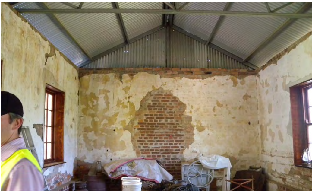
Figure 27 The interior of the barn showing the original walls, new roof structure and new windows in original openings. Source: Paul Davies Pty Ltd November 2009.
