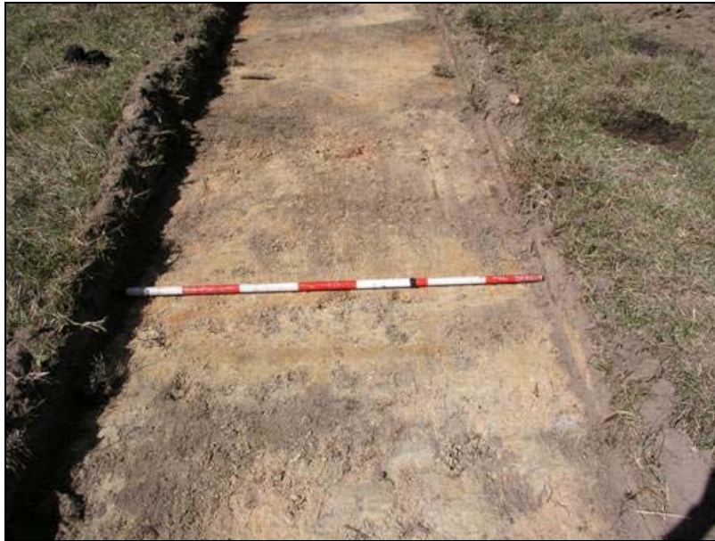
Figure 32: Example of excavation techniques - Front Paddock Trench 8
