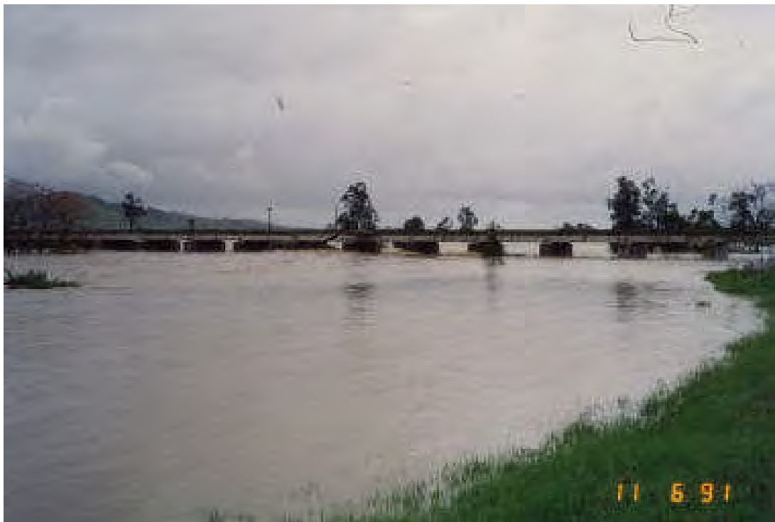
2..US RAIL BRIDGE (Note afflux above central spans
