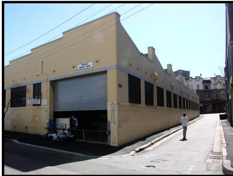
Figure 31: Depiction of the Hart and Hudson Street façades showing the saw tooth roof which creates a stepped skyline at the rear of the building. Note also the original 12 pane, metal frame windows. (Source: Photography by Rappoport Pty Ltd, August 2008).
