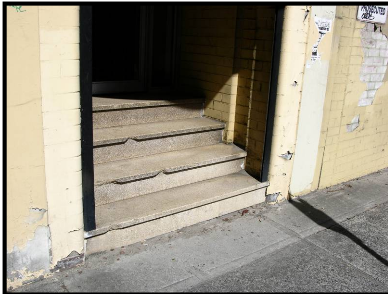
Figure 33: Depiction of the original terrazzo steps at the Cleveland Street entry. (Source: Photography by Rappoport Pty Ltd, August 2008).
