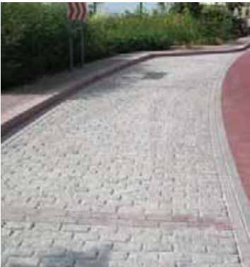
road pavement in coloured concrete with patterning in cobbles
