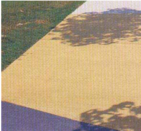
broom finished path with key nodes defined in exposed aggregate concrete or panels of full depth coloured concrete
