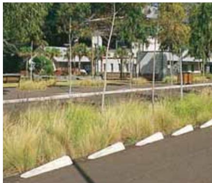
feature bollards or similar barrier to restrict access into planted swale
