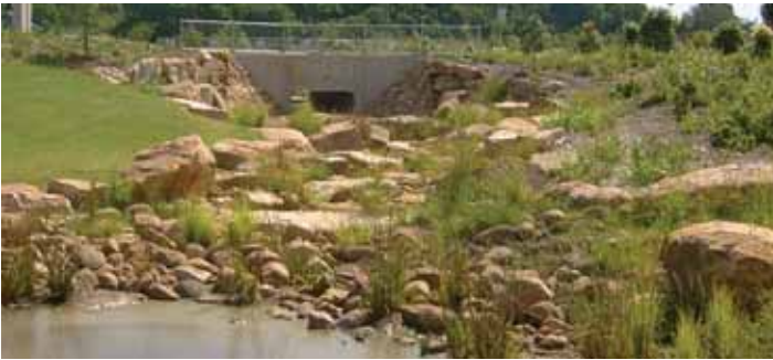
stormwater outlet with planting & rocks
