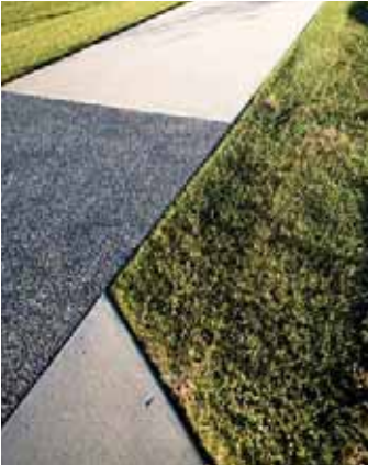
broom finished path with key nodes defined in exposed aggregate concrete or panels of full depth coloured concrete
