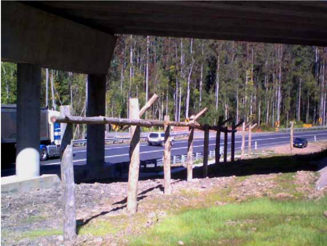
Photograph 1. Koala-friendly structures to encourage movement through this underpass, Pacific Highway Reconstruction, Bonville (Photograph, S. Cotter)
