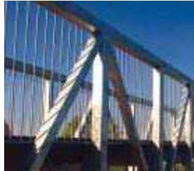
steel frame & recycled plastic decking to bridge
