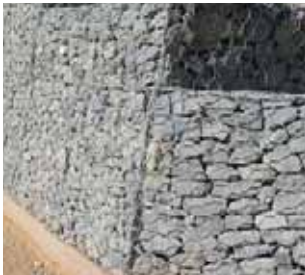
gabion rock retaining walls
