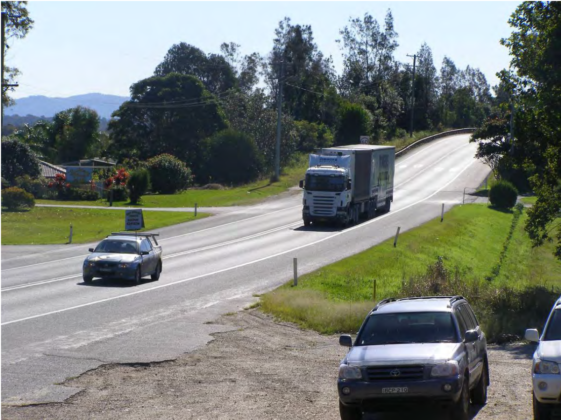
Plate 2.3 View of the existing access to the Site looking north
