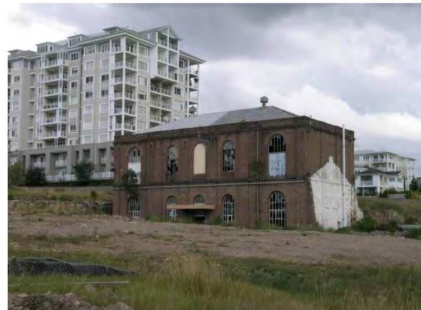
The Plumbers' Workshop
