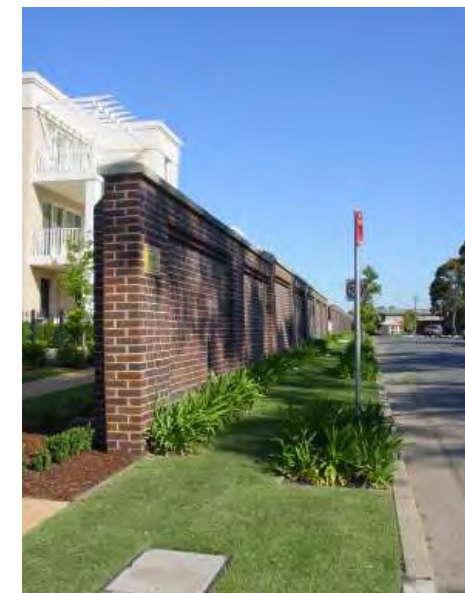
Tennyson Rd Wall
